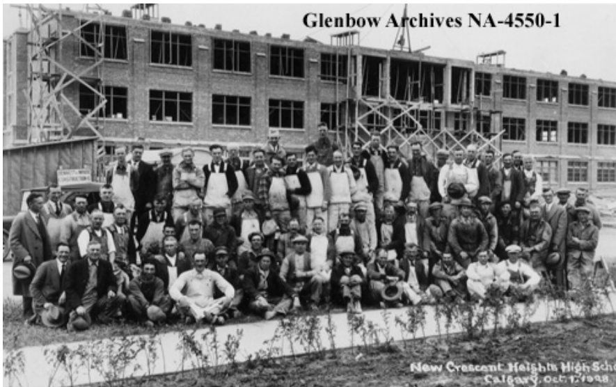
Construction crew at new Crescent Heights High School, October 1, 1928. Glenbow Archives, NA-4550-1.
