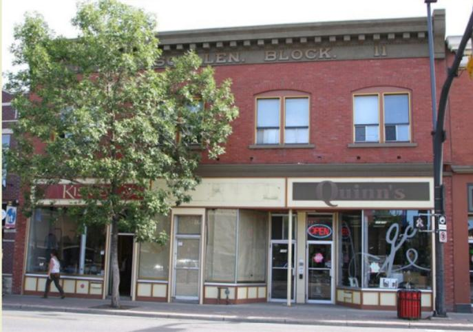
All of these were lost in a 1966 renovation in which the facade was covered with aluminum siding, the cornice removed, and the windows and storefronts entirely changed.
