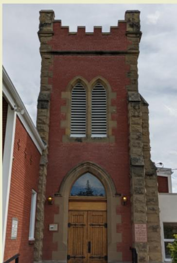
The brick and stone English-style church building burned in January 1957, leaving only the tower. It was replaced the following year by a new brick church. The rock-faced sandstone is articulated by horizontal string courses at the levels of the sills and lintels. A classic balustrade is supported by columns over the entrance; the balustrades which used to sit atop the cornice everywhere but in the centre have disappeared.
