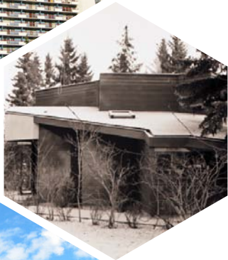
LEAVITT RESIDENCE 920 Prospect Avenue SW 1970 Gordon Atkins
