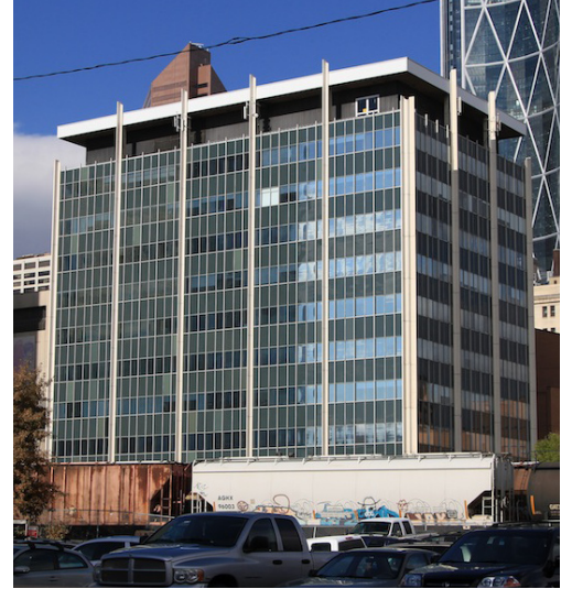
NATURAL RESOURCES BUILDING 205 9TH AVE. SE
