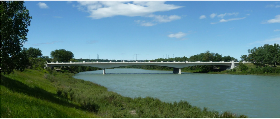
MEWATA BRIDGE, 14TH STREET SW
