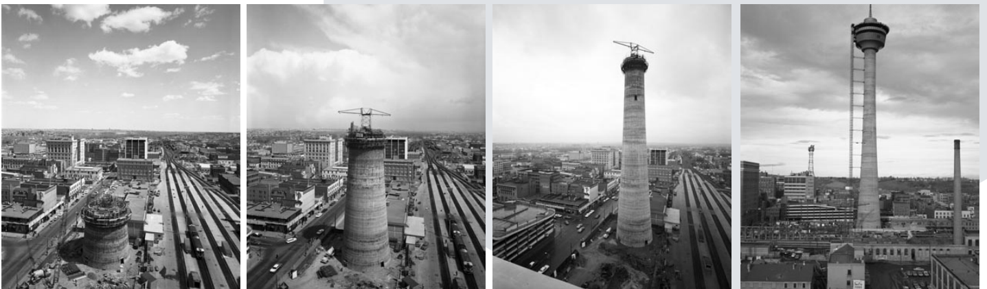
BUILDING THE CALGARY TOWER, 1967 GLENBOW ARCHIVES
