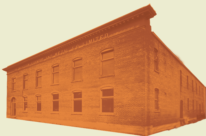
Western Steel Products Plant (pg 11)
