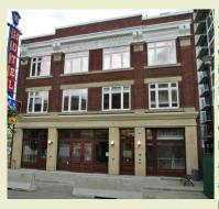
The exterior character-defining elements of the St. Louis Hotel include such features as its: three-storey, rectangular plan with short façade and flat roof; brick and tile construction; açade brickwork laid in stretcher bond with raked joints, and articulated to create pilasters and panels, and forming a straight parapet, and illuminated 1950s signage suspended from the facade.
