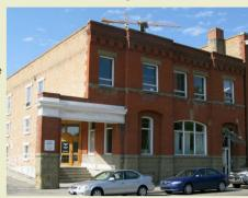
The building is defined by its two-storey, rectangular, flat-roof form with asymmetrical facade; raised basement and ground floor, heavy-timber construction with brick exterior; red, pressed-brick facade with heavily corbelled cornice; battered rock-faced sandstone foundation rock-faced sandstone sill course, window sills and lintels.
