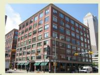
at the time of its construction. It features reinforced concrete floors, slab and beams, with steel frame window openings and solid brick walls. Bays of large windows with concrete lintels are set between vertical brick piers, which define the overall look of the façade and serve to express the building's internal structure.
